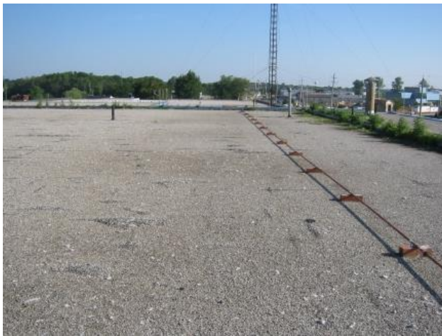
Roof Surface as seen during day
